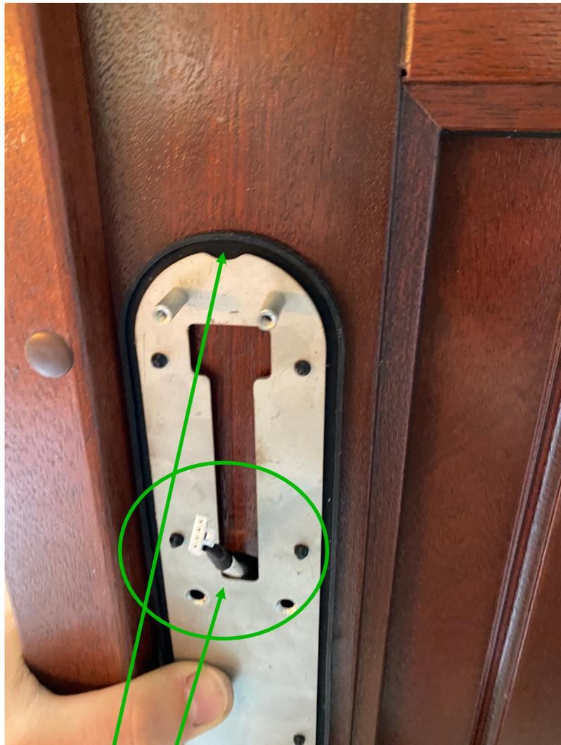
Make sure the rubber plate is installed and that the cable is through to connect with the back panel.
