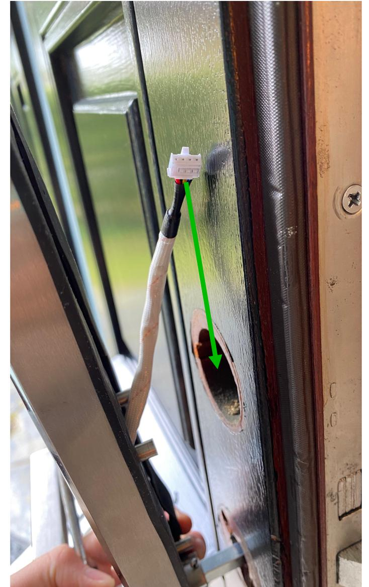
! The cable needs to get through this hole in the mortise lock to connect with the back panel !
