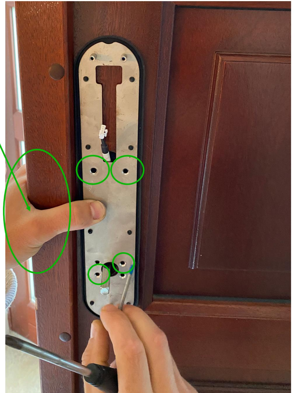
**XLOCK TIP:** In some cases the screws need to be adjusted to the thickness of the door. The screws can be cut with a metal saw.
